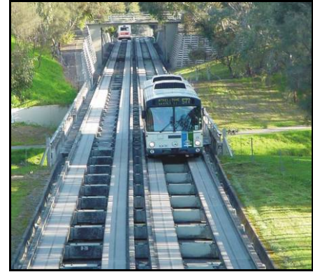
Bus in Guideway
